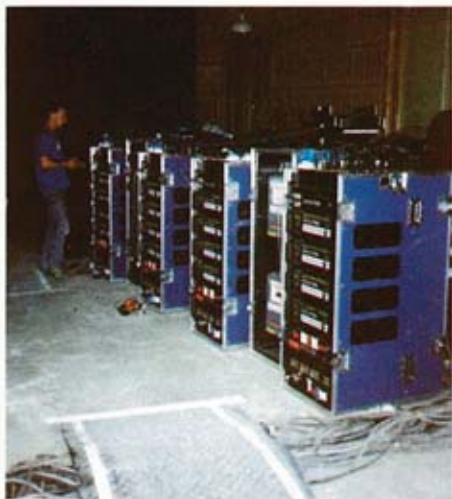
Adam Bennett, R+D engineer with the four TV dimming systems in the gallery of the Royal Albert Hall
