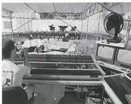
Meteorlites' stage lighting control set-up using a Celco Gold and 30 Major.
