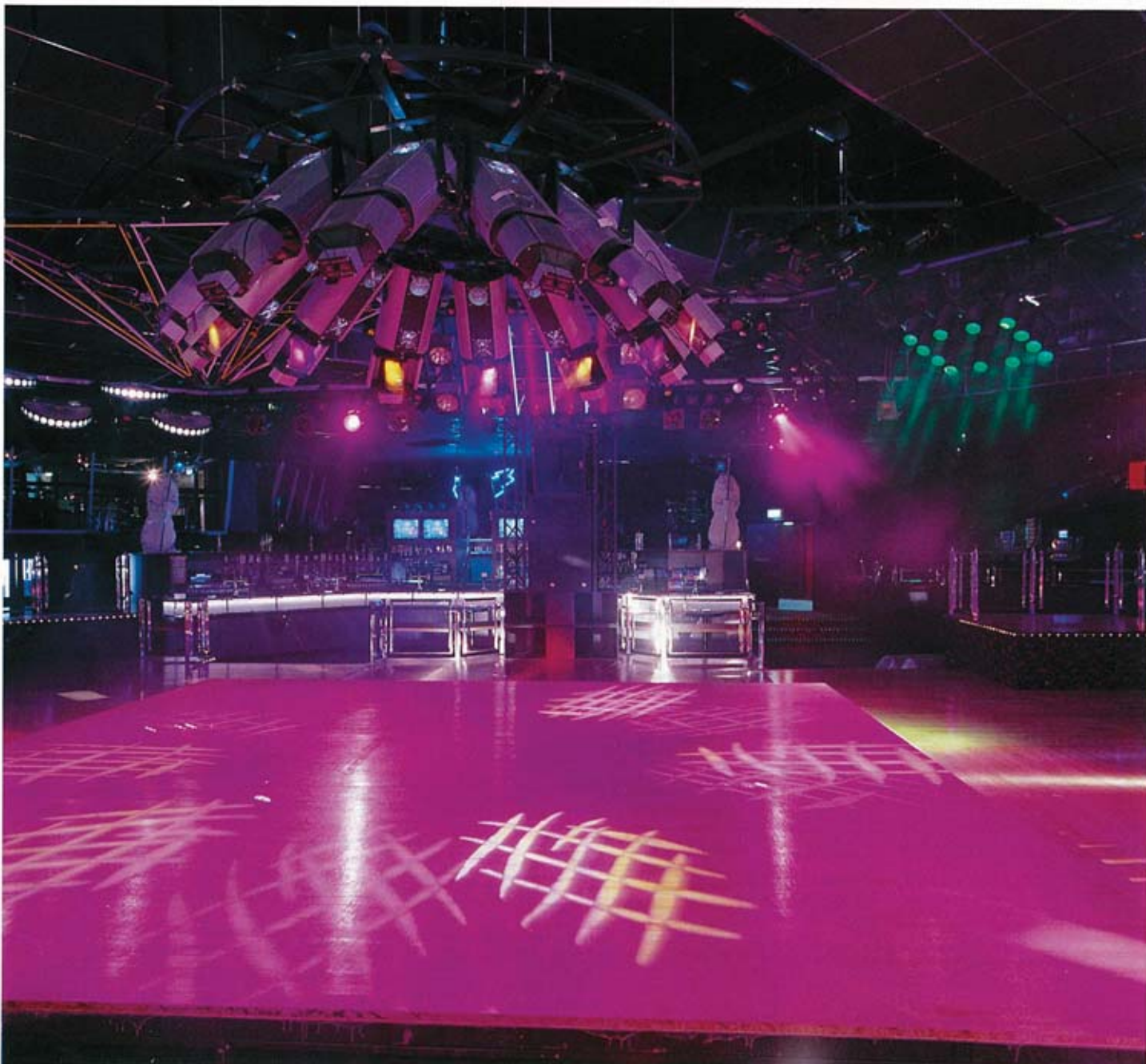
The cluster of Golden Scans replaces the central speaker array at the previous venue.
